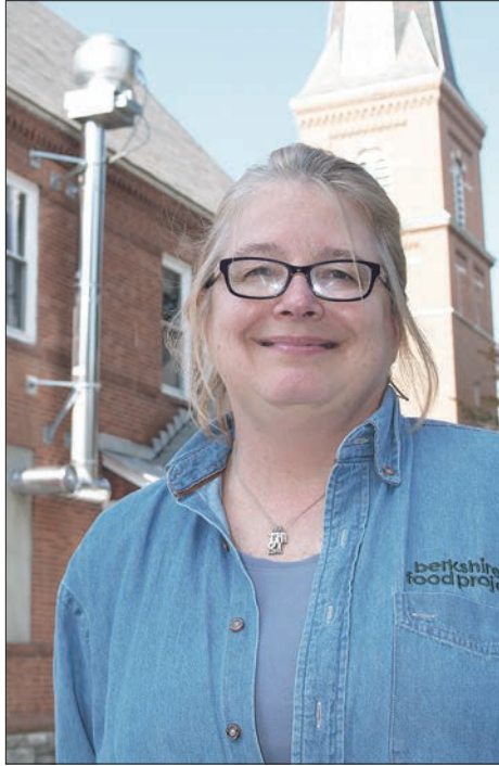
Kim McMann, executive director of the Berkshire Food Project, stands by the new exhaust system installed as part of a major renovation of the kitchen the organization uses within the First Congregational Church in North Adams.
